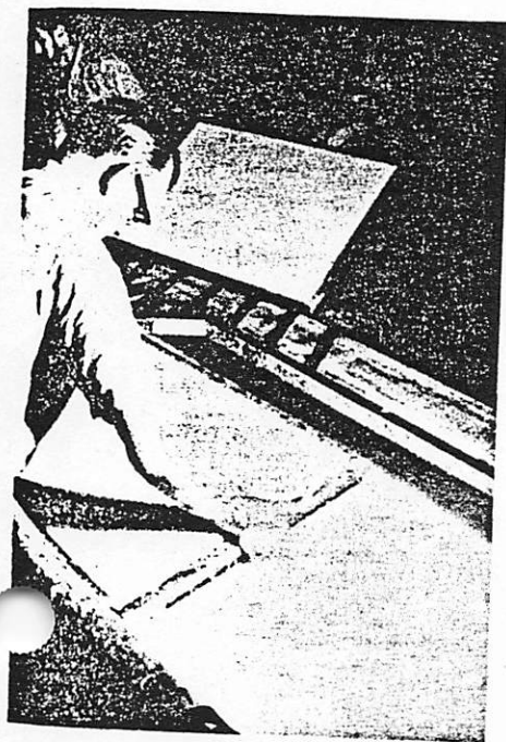
3. Vatman lifting mold out of vat, J. Barcham Green, Ltd., Kent, England
